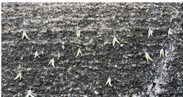
Figure 7. Young ball moss attached to outside of a building wall.
